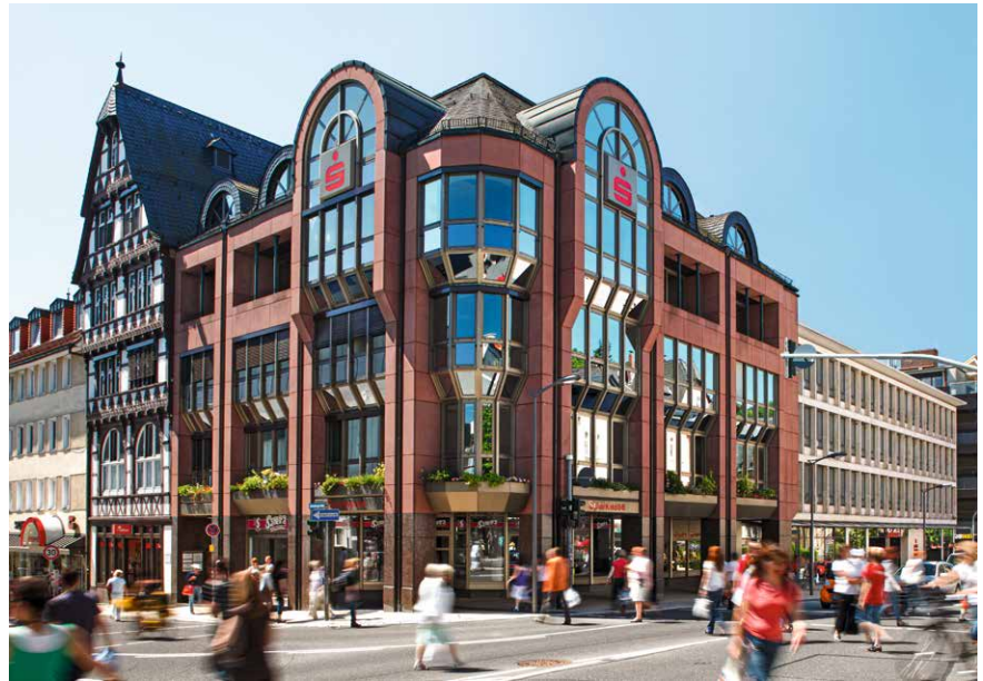
Main branch of the Sparkasse in Marburg
