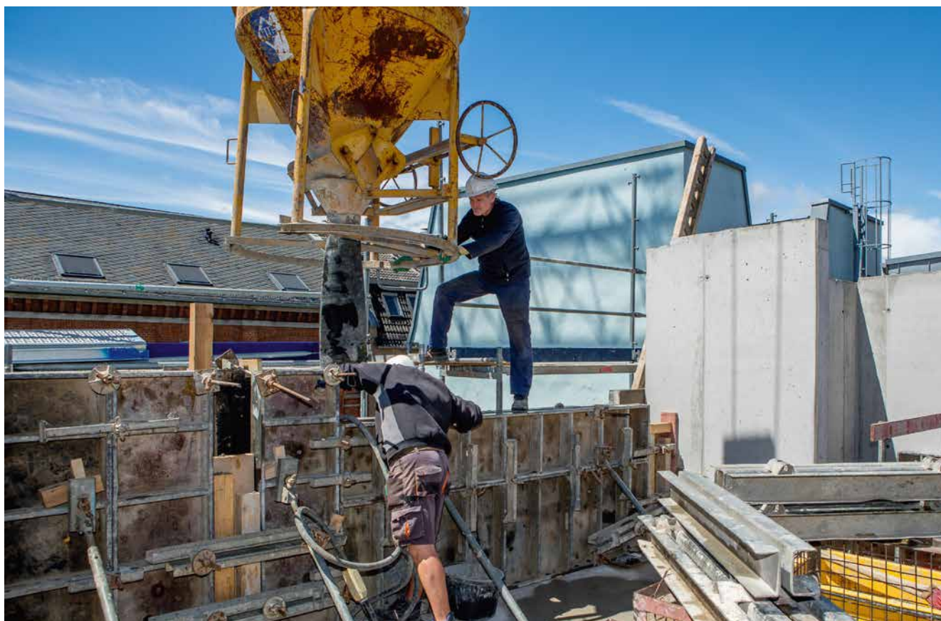
High-precision work: On the roof terraces of the town houses, the last remaining walls are filled with liquid concrete.
